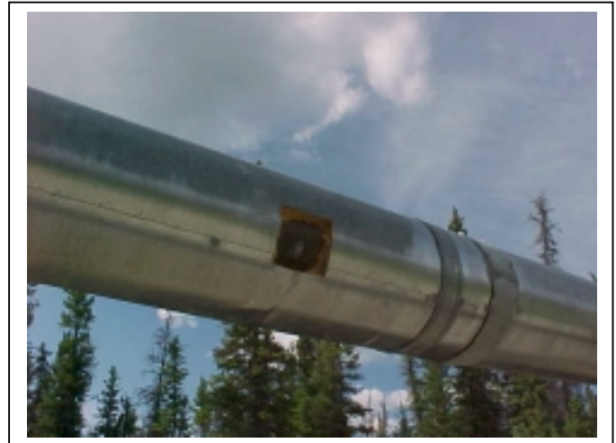
In the first week of the maintenance project, an inattentive equipment operator struck the pipeline with a backhoe bucket. Here Alyeska has removed the sheath and insulation to check the condition of the pipeline itself. No damage was found.
